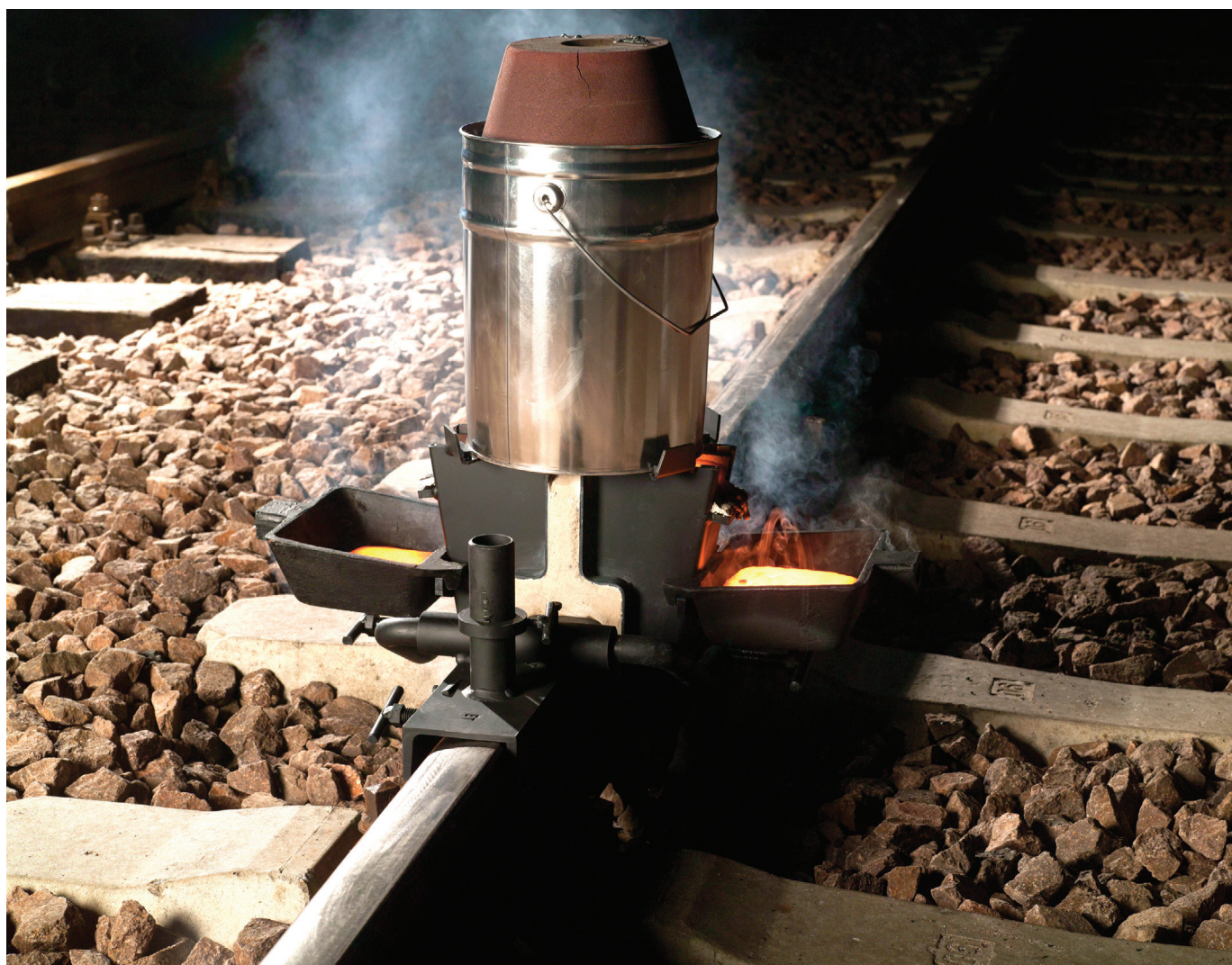
Aluminothermic welding might look old fashioned but it is a process that has evolved over time and remains extremely effective.
