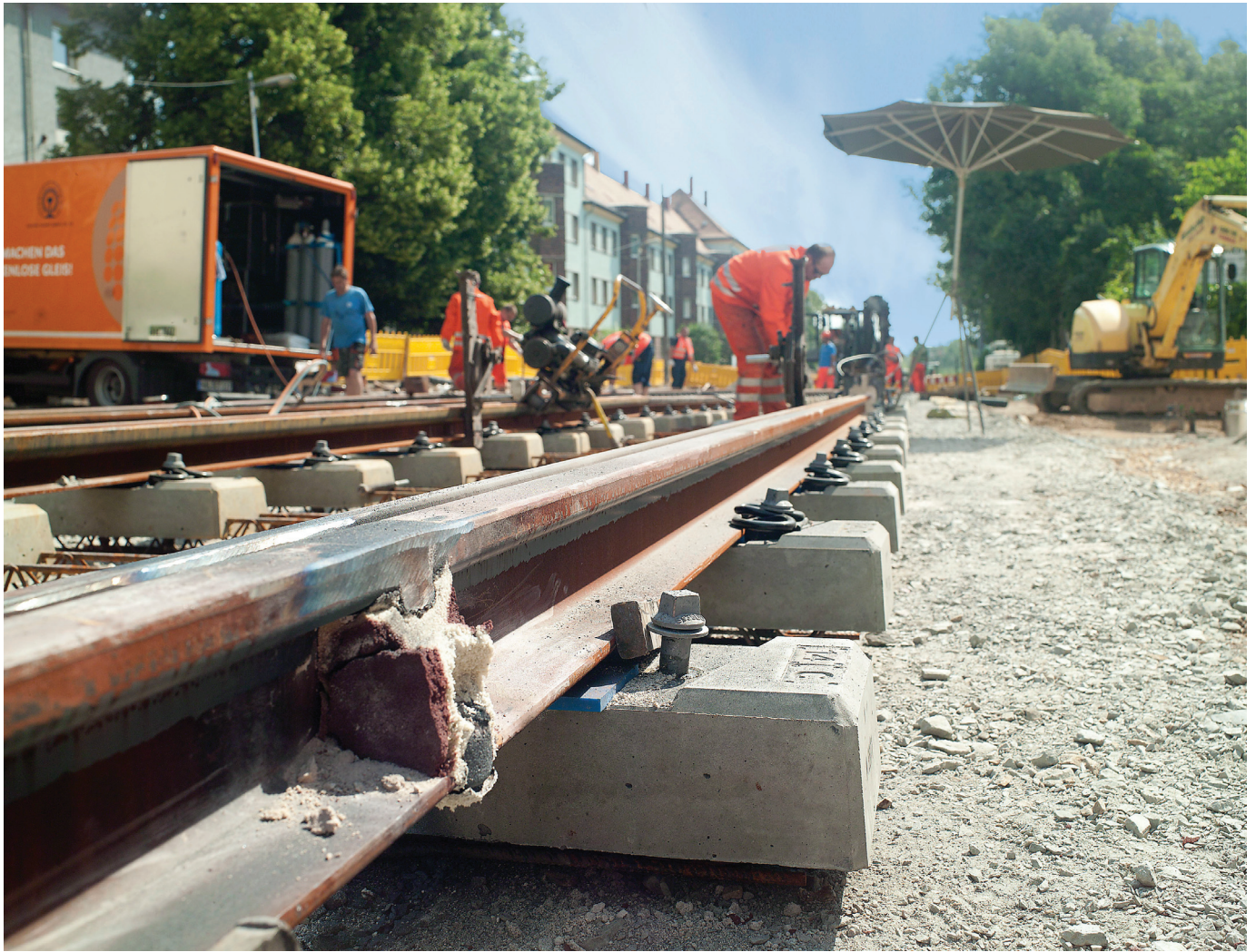
Welding grooved rails for light rail applications has proved challenging with no European Standard yet established for this process.
