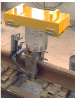
Figure 3: Placing the Envirofilter™ parallel to the rail
