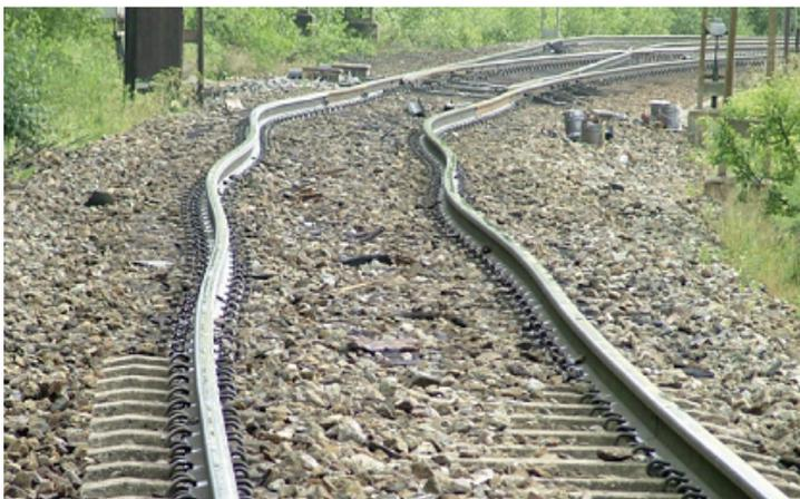
Fig. 1: Picture of a transverse buckle near a switch due to inadmissible high longitudinal compressive load stresses resulting in a ballast resistance stability problem. In contrast to regular curves, often allowing a certain transverse displacement reducing the peak amplitude of compressive stress, the switch can act as a fixed point in the curve. The compressive stress enters the buckling regime, then finally exceeds the strength against transverse track buckling.
