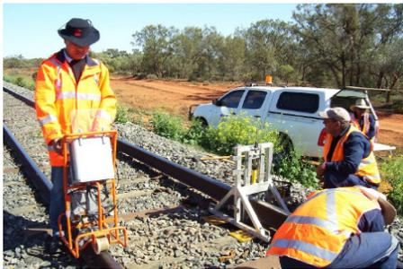
Fig. 5: Picture of a trial in Broken Hill, Australia. On an A.R.T.C railway line comparative as well as supplementary measurements between RAILSCAN and A-frame SFT equipment were performed in order to study not only the capability of the two methods but also the possibilities of increasing the SFT inspection performance in different situations under different random conditions. Attention also has been paid to SFT measurement in narrow curves & sections with decreased ballast density.
