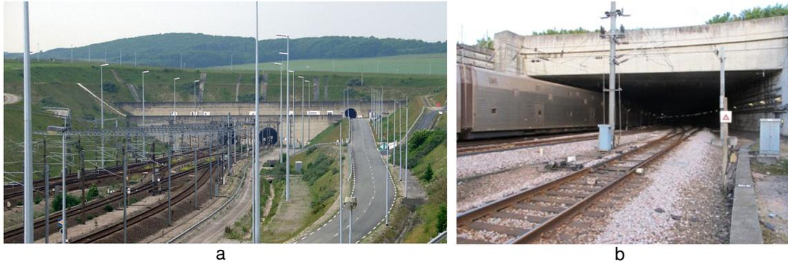
Fig. 4: RAILSCAN SFT inspections in the EUROTUNNEL Calais-Folkestone. a: Underground twin tube tunnel portal at the French side near Calais. b: Terminal loops with above ground tunnel on the UK side at Folkestone.
