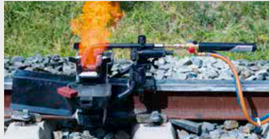
Preheating with the Smartweld Record device.
